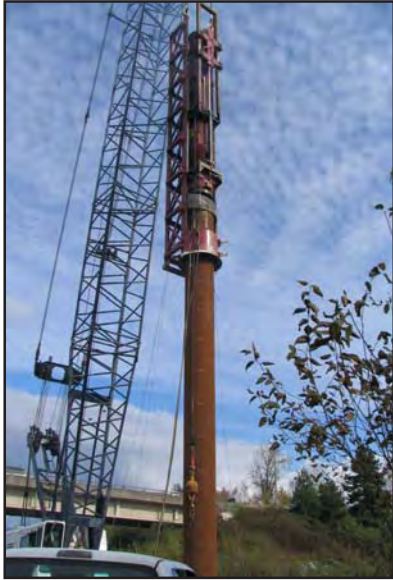
D180-42 driving 48" piles with a 54" offshore.
